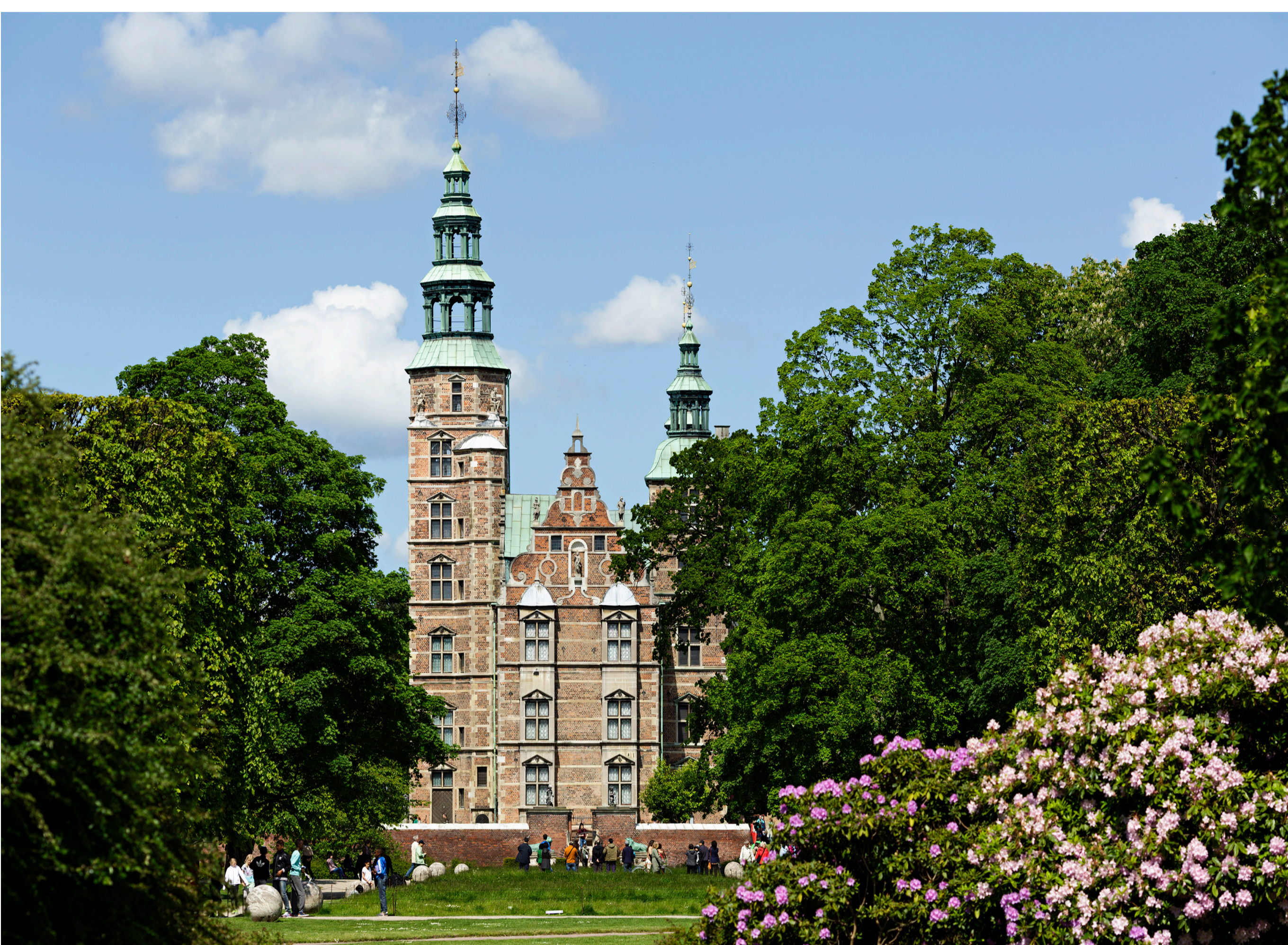
Fig. 1 – Main facade of Rosenberg Castle, Copenhagen, Denmark.
